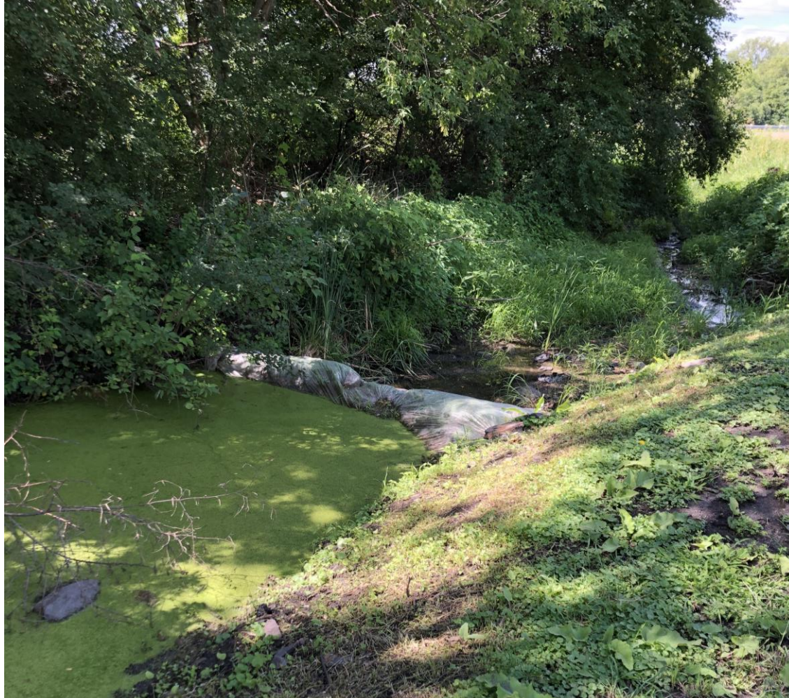
Figure 3 Rock Water Level Control Structure
